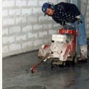
6) Next step in producing monolithic industrial floor is cutting construction and shrinkage joints.
