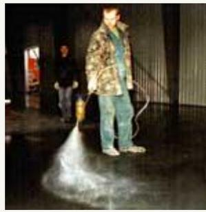
5) Immediately after finishing, spray apply BAUSEAL ENDURO-acrylic sealer to the surface to give curing and sealing treatment to the floor.
