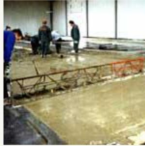
1) Concrete should be laid down and compacted with a specially designed precision engineered vibrating screed which allows to vibrate the concrete up to 30 cm of depth. Vibration can be adjusted according to the slump of the concrete.
