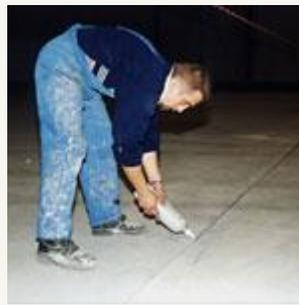
7) The final step is treating construction and shrinkage joints with BAUFLEX JOINT SEALANT SYSTEM.
