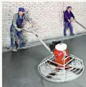
3) When the concrete can just take the weight of an operator leaving a slight imprint on the surface we can start to power float. To achieve best monolithic result, first power floating must be done by using (disc, pan) followed by finishing by repeated passes of a power trowel with blades until a flat hard and shiny finish is produced.
