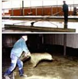
2) When an automatic spreader is used in conjunction with a laser screed, Dry Shakes are spread evenly onto the concrete immediately after screeding. With a manual application Dry Shakes should be sprinkled onto the screeded concrete in 2 stages. In both cases each application of Hardener should be leveled and worked into the concrete using a BUMP CUTTER SCREED.
