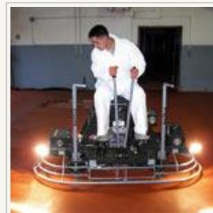
4) Final finishing to close pores and remove undulations can be achieved either by walk behind trowel or riding trowel.
