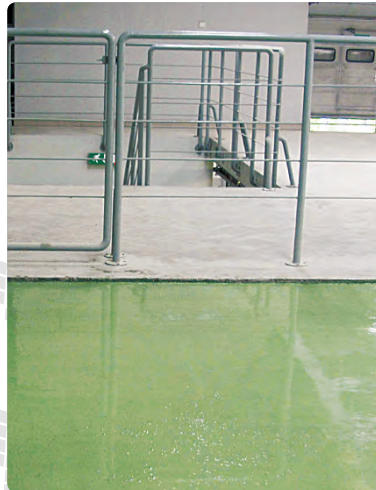
BAUFLOOR® rolled – "orange peel" effect
